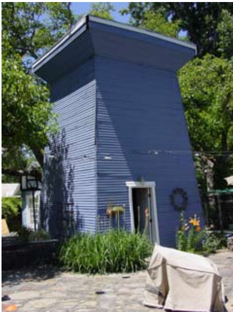
WATERTOWER BEHIND HOUSE
